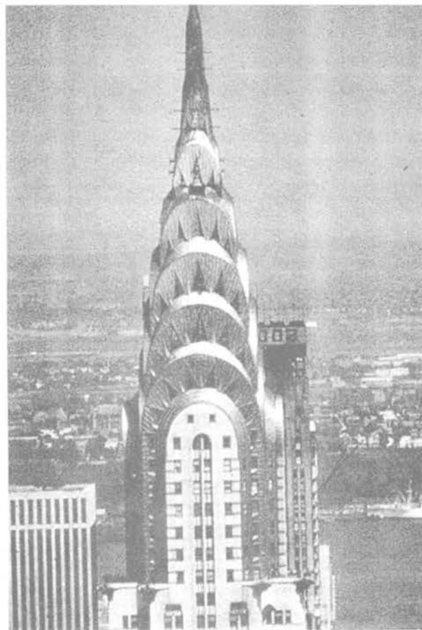
Fig 11. Stainless steel cladding dating from 1929; Chrysler Building, New York
